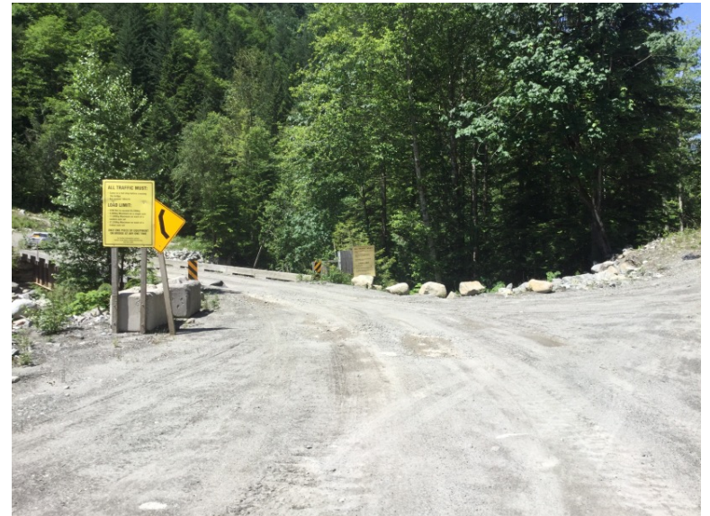
Approach from Right Bank when facing downstream
