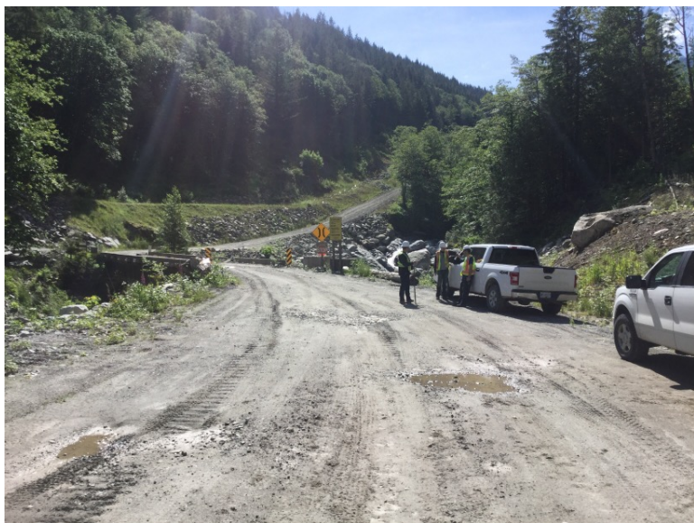
Approach from Left Bank when facing downstream
