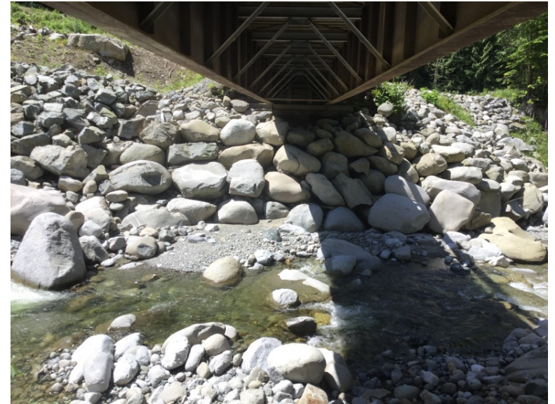
Left Bank Abutment when facing downstream
