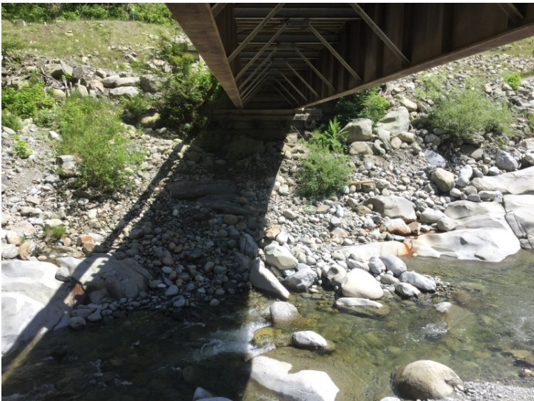
Right Bank Abutment when facing downstream
